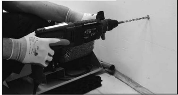
After marking the drill holes, place the shoe polishing machine on a rubber mat with two persons. Use a suitable electric drilling machine and a masonry drill bit (diam. 10 mm) to drill holes at the previously defined four marks using an 85 mm depth stop. After drilling the holes use a suitable suction unit to clean the holes and press in flush dowel pins 10 mm supplied into the respective boreholes.
